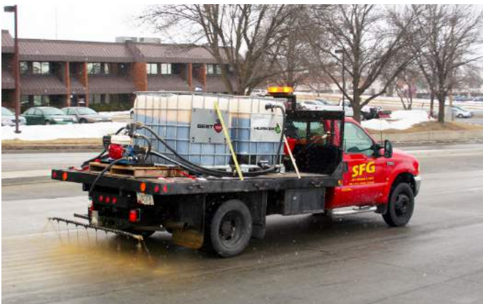
Applying Husker Plus RTU
